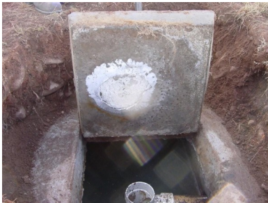
Note the etching of the lid directly above the T-Baffle in the photo above, and the corrosion of the D-Box sidewall in the photo below.
