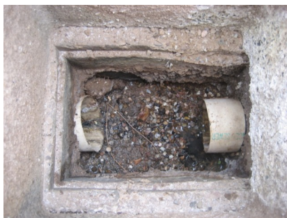
Note the etching of the lid directly above the T-Baffle in the photo above, and the corrosion of the D-Box sidewall in the photo below.
